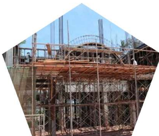
Constructions of Seeduwa building complex
